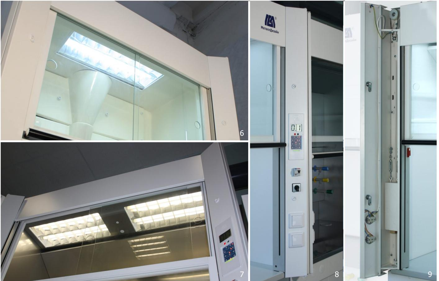
to provide a uniform motion of the sliding screen. The weight is located in the left column of the portal (Pic. 9). All parts (weight, cable in polyethylene housing, rollers) are accessible for maintenance and repair directly from the front side of the hood. It is particularly important if the hood is located in a corner of the room or situated in a single row with other exhaust hoods.
