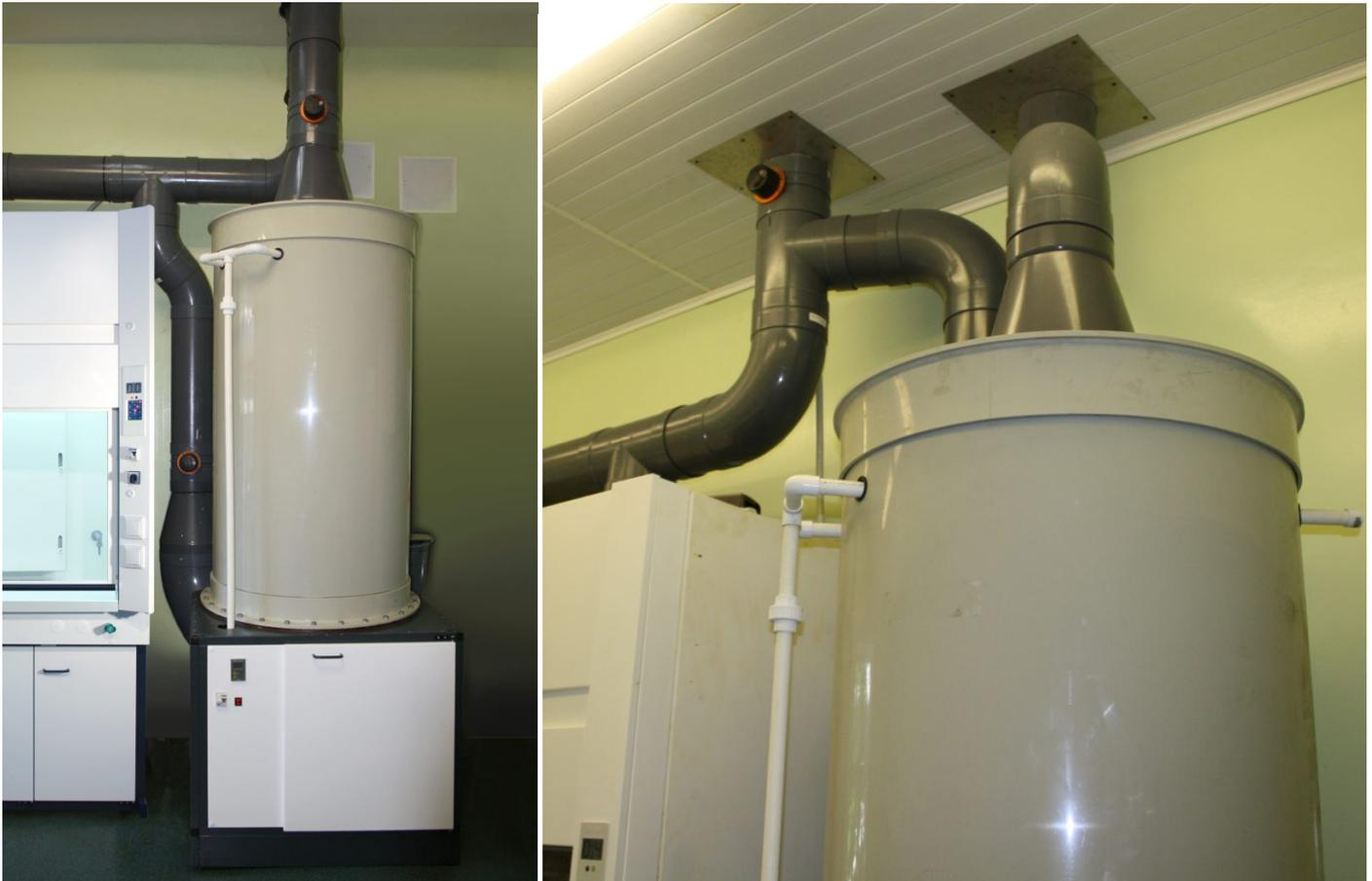
The scrubber is designed for recovery acids vapor in the air flow coming out of exhaust hoods in laboratories.
